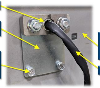
Conveyor frames must be bonded together and connected to earth ground at a single point
