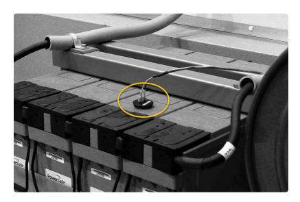
The probe senses battery temperature variation and adjusts output float/equalize voltages to compensate. If battery temperature increases, ATevo's output voltage decreases. If you are experiencing any inconsistencies in ATevo when the probe is installed, temporarily disable the TempCo Option per Section 4.11.
