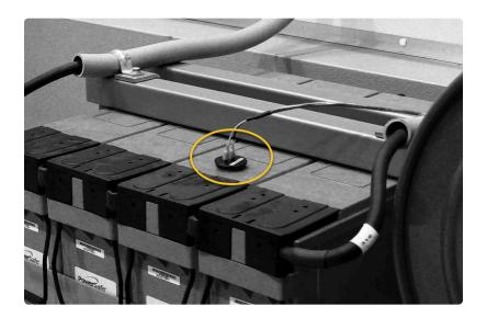
The TempCo probe (A10), or 'puck', is the same for all battery types and all ATevo models, regardless of dc output voltage. TempCo accessory kits (p/n EJ5304-##) differ, depending on cable length (25ft, 50ft, 100ft, etc.).
